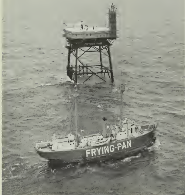
REPLACEMENT —Coast Guard light tower off Cape Fear, N.C. replaces 34-year-old lightship at Frying Pan Shoals.
